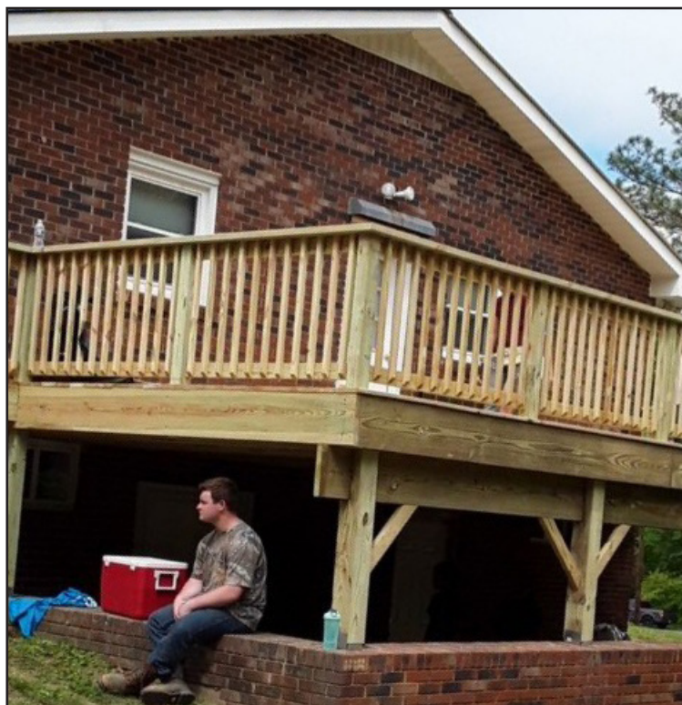
LEWIS UNIVERSITY HABITAT FOR HUMANITY
